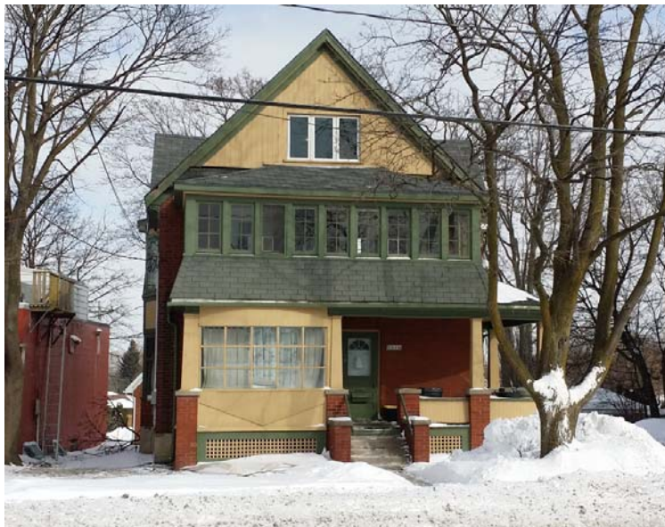
Single family home converted to four-plex at 1510 King St. E. in Kitchener
